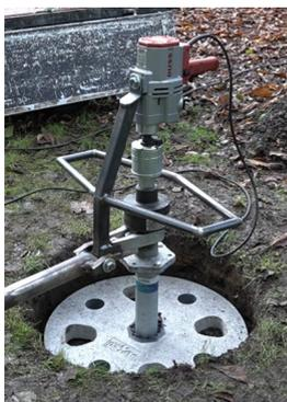
In addition to elevated pile loads, the paXos RFS can also be used for **building loads (BL)**, e.g. to base containers or prefabricated buildings. In this case, a special attachment distributes the weight load ideally over the precast concrete slab, allowing up to **16 tons of load** per foundation slab to be absorbed.
